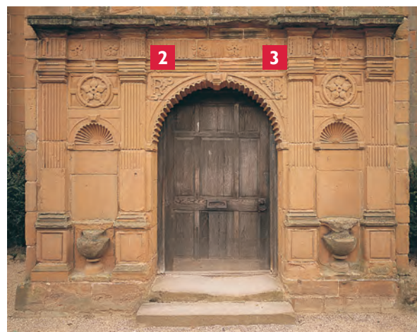
The entrance doorway of Leicester's Gatehouse.
