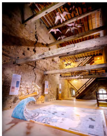
The second floor of the keep.
