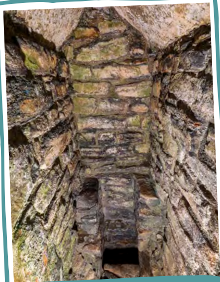
The inside of the latrine and its chute in the east curtain wall at Richmond Castle.
